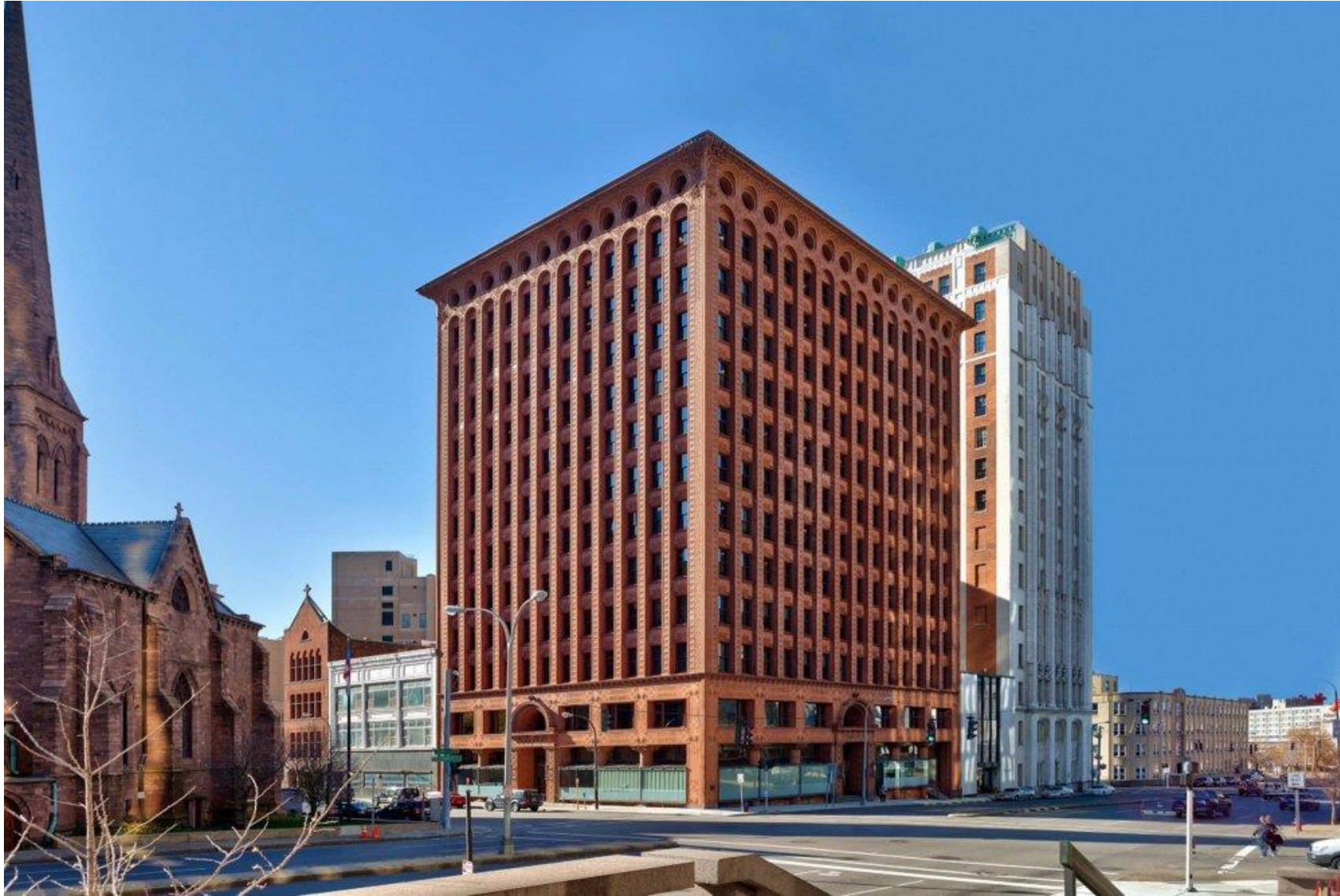
Prudential (Guaranty) Building, Buffalo (Louis Sullivan, Dankmar Adler), 1896 Copyright: Gene Avallone (M/E Engineering)
